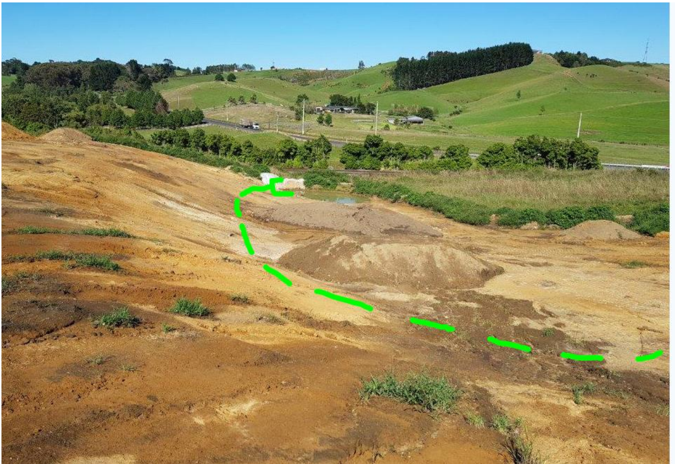
Requested underfill drain in green.
